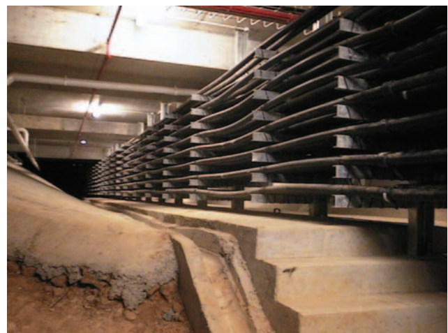
Fig. 2. View from underneath the Geoscience Australia building showing pipes circulating water between the pump room and the underground bore field.
