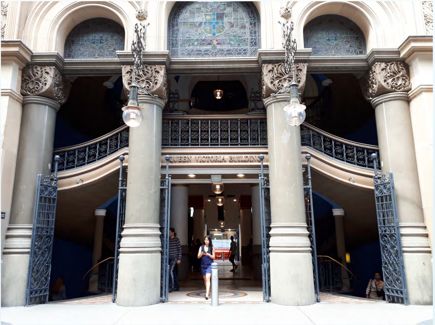
Polished columns of Bowral Trachyte at the western entrance to the Queen Victoria Building in Sydney. There are 75 columns of Bowral Trachyte which support rows of arches around the building. See www.visitsydneyaustralia.com.au/queen-vic-bldg.html . Photo courtesy Mike Smith.
